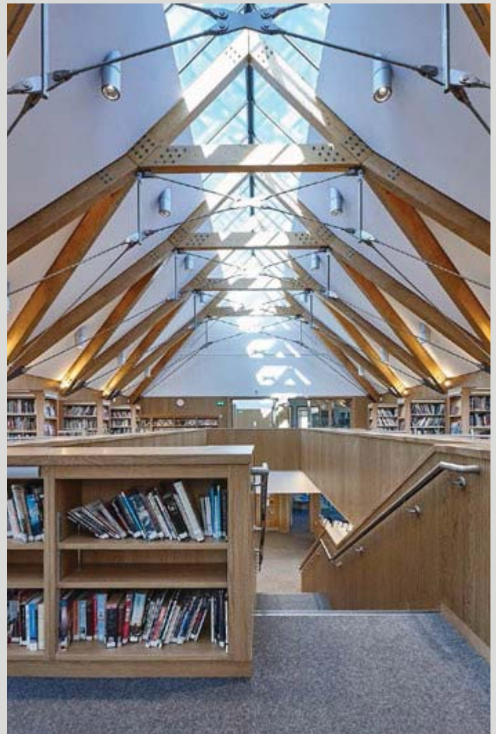
Library - UNITED KINGDOM Acoustic ceiling Installation: ACOUSTIC GRG
