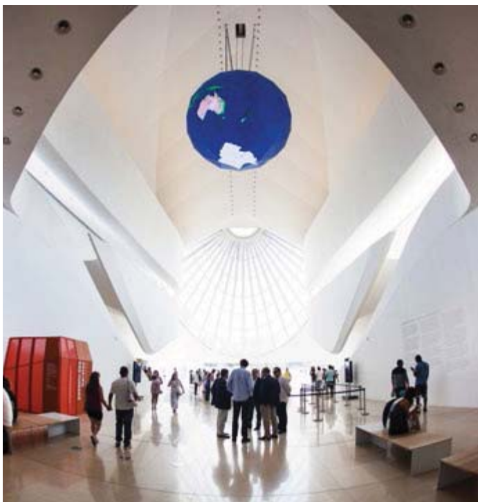
Museum of Tomorrow - Rio - BRAZIL Ceiling and crawling dressings in white acoustic fabric Architect: Santiago Calatrava - Installation: DIARCO Ltda.
